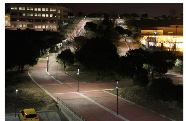
BAT-Street Lighting technology - UPM-Open-IoT
